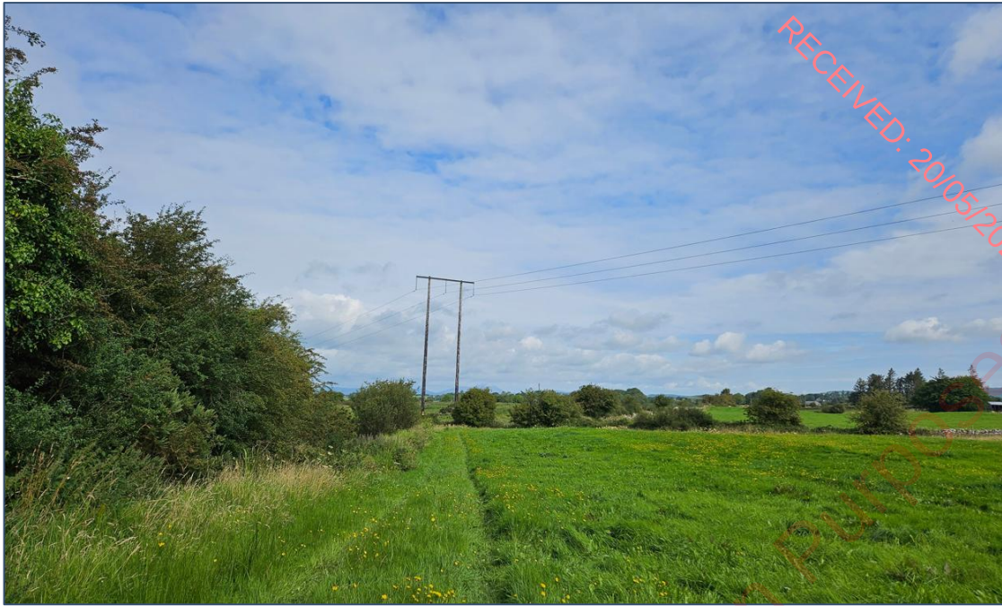
Plate 13-18 Location of the western-most end mast at the north-west of the Site in an agricultural field lined with vegetation.
